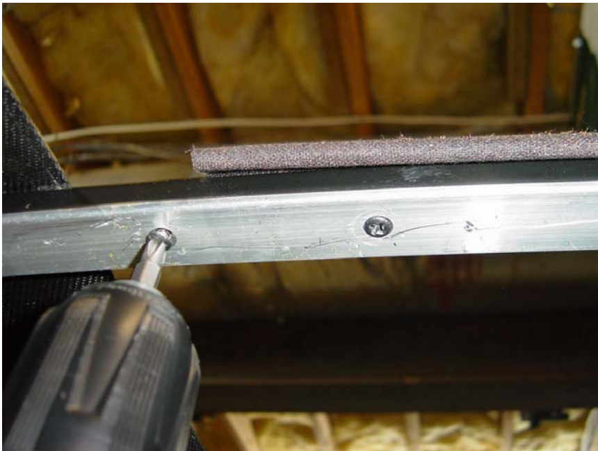
Figure 18: Removing aluminum strips that hold top fabric to second and third bows.
